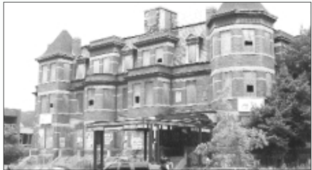
photo—Paul K. Williams, June 6, 2002. The severely dilapidated and abandoned state of the four homes formerly occupied by Hines attracts homeless people and vagrants to dwell under its protective covering day and night.
