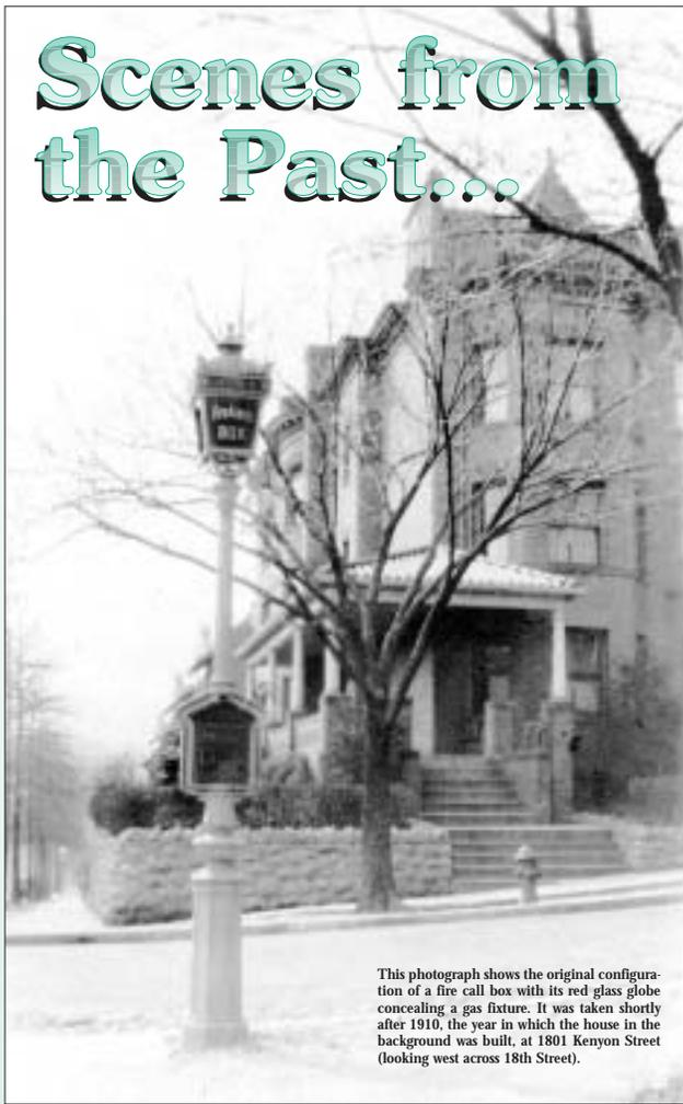
This photograph shows the original configuration of a fire call box with its red glass globe concealing a gas fixture. It was taken shortly after 1910, the year in which the house in the background was built, at 1801 Kenyon Street (looking west across 18th Street).
